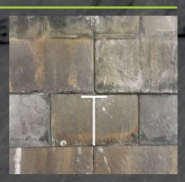
To conclude the line drawings for cutting purposes, measure 37.5mm / 1.48" left and right from the centre of the rafter line. Draw vertical lines from the 190mm / 7.5" horizontal line, down to the bottom of the slate.
