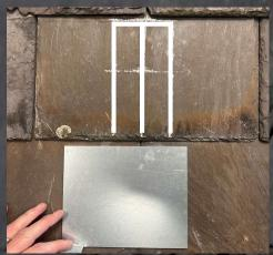
5 Insert the SpeedFlash® Shield fully as shown.
