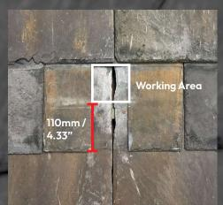
7 Using the angle grinder, cut out the 'working area' on the slate i.e. the area from the 110mm / 4.33" horizontal line and the 190mm/7.5" horizontal line.
