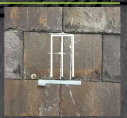
6 Now you have cut the top slate(s), you need to cut the lower course to create the working area (the area in which the bracket will be fixed).
